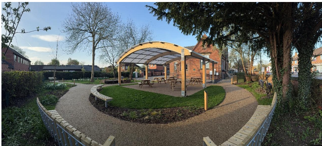
Works completed in December 2025
